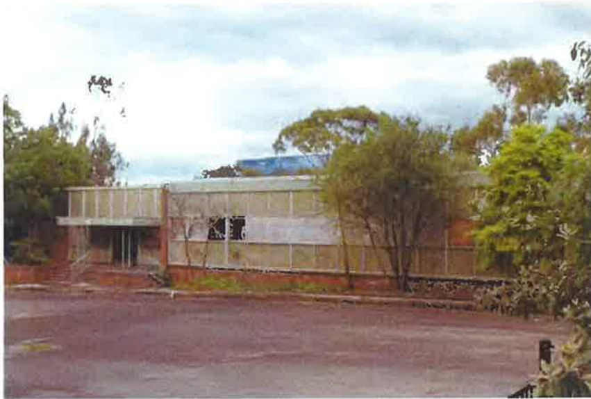
Figure 3 – Existing building at the site
